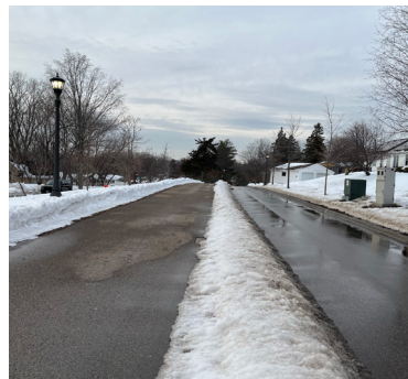
Wheelock Parkway - Saint Paul Separated trail, snow storage between bike facility and roadway
