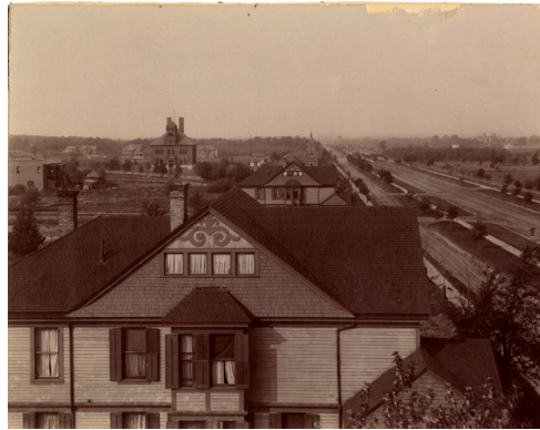
Figure 5. View of Summit Avenue from rooftop, looking northwest, c. 1900.
