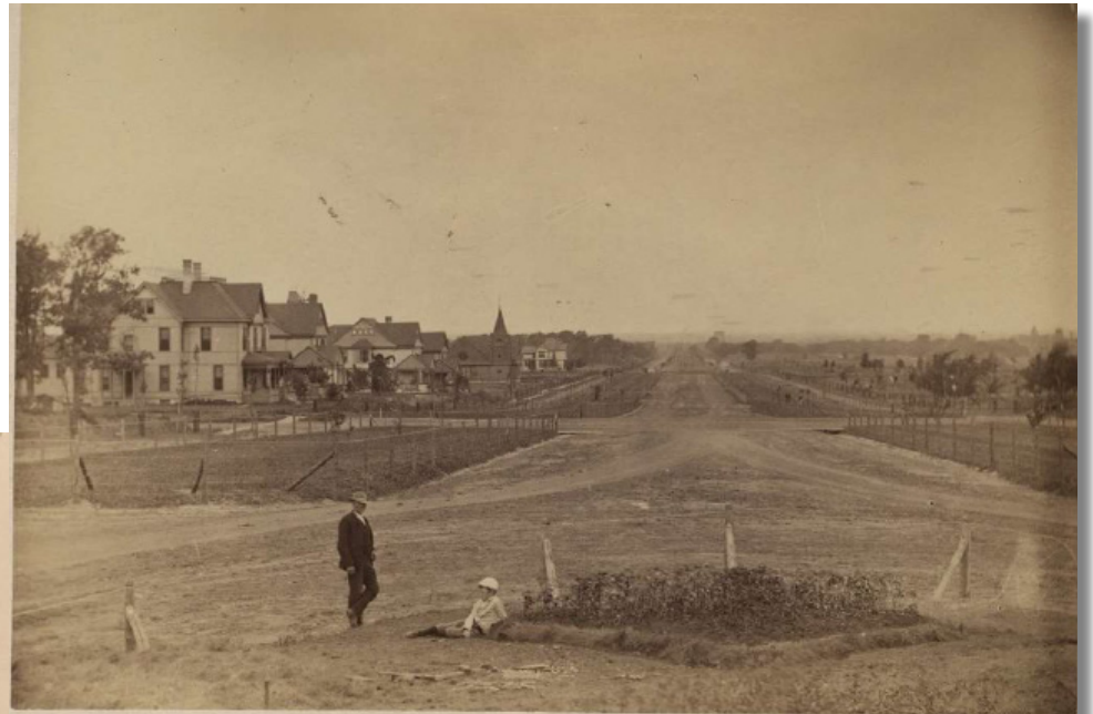
View of Summit Avenue near Macalester College, looking west, 1890 Credit: Minnesota Historical Society
