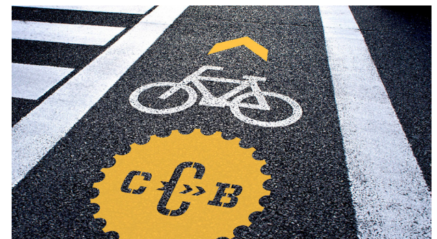
Example: Wayfinding on Capital City Bikeway
