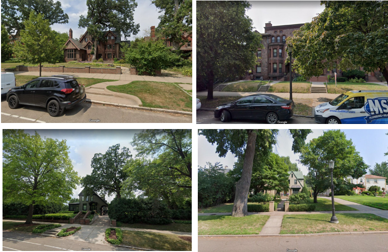
Figure 5: Retaining walls, concrete stairs, and planting beds about the right-of-way along Summit Avenue
