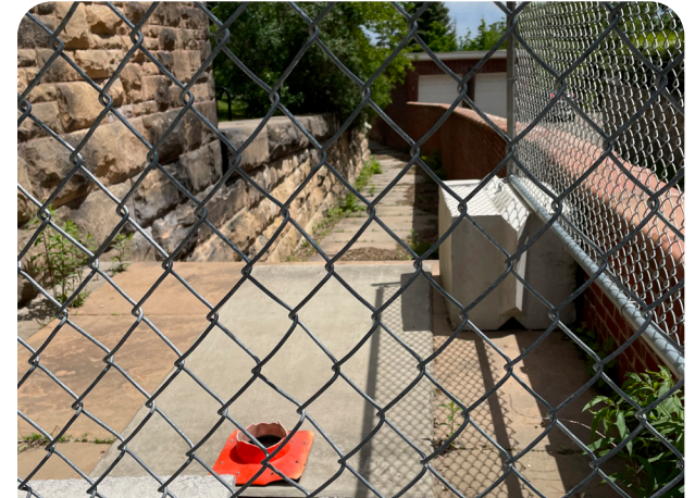
No access to Walnut Street steps, a potential connection point
