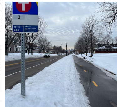
Como Avenue - Saint Paul Separated trail, snow storage between bike facility and roadway
